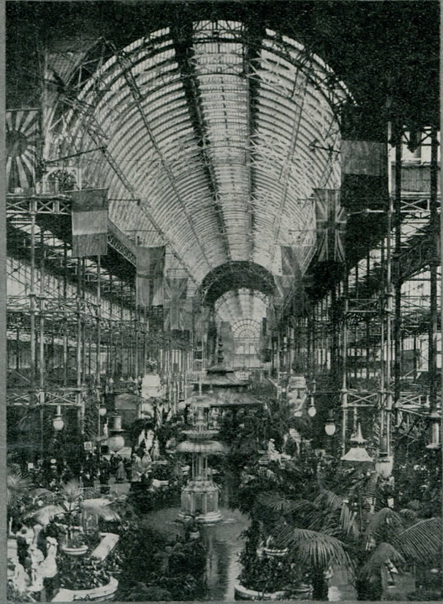
CENTRE TRANSEPT, SOUTH NAVE.
